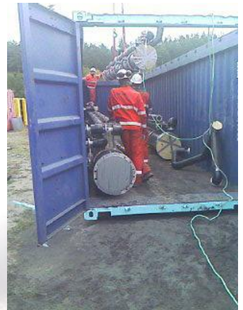
Unloading a 13 ton pre-insulated steel pipe in Norway
